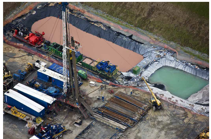
Well pad during drilling process in Dimock, PA Source: J Henry Fair
